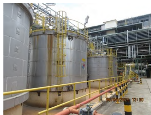
Stripped wastewater tank
